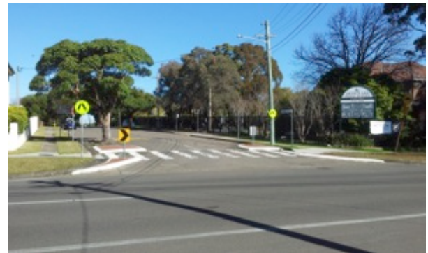
Noble St, Concord: Pedestrian priority through crossing and tree and kerb blister to narrow Rd
