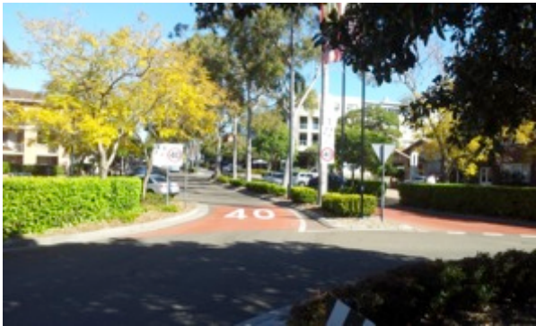
Majors Bay Rd, Concord: landscaped kerb extensions, effective roundabout and 40km/h zoning
