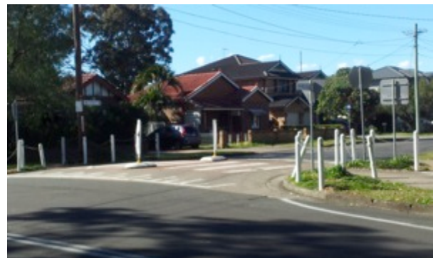
Archer St, Concord: Pedestrian priority through crossing and post and kerb blister to narrow Rd and indicate a residential area.
